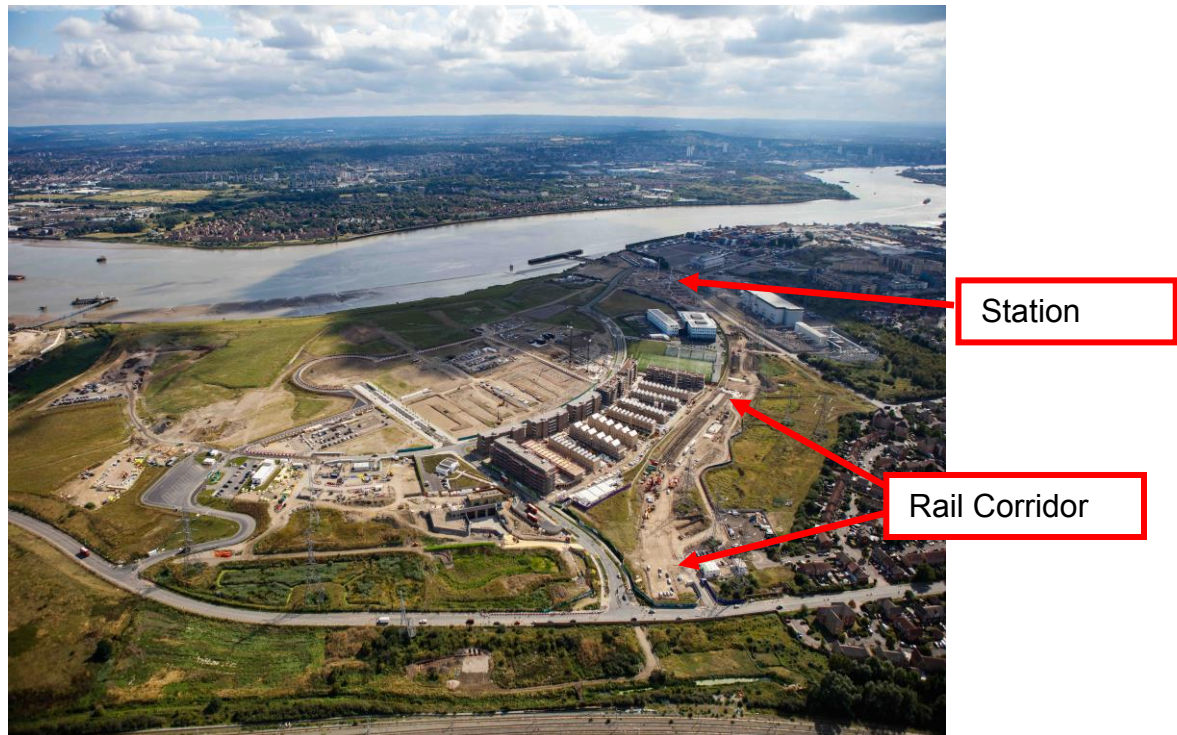
Fig 2: Barking Riverside Development September 2019 – rail corridor taking shape
